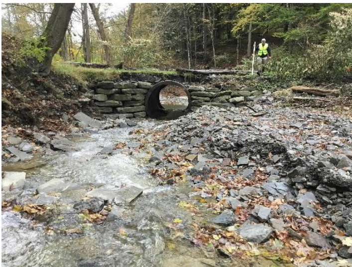
Private Driveway off Dean Street over Huntington Creek (upstream). Structure inlet. Note erosion of road along top of structure, and sediment deposition on river right.
