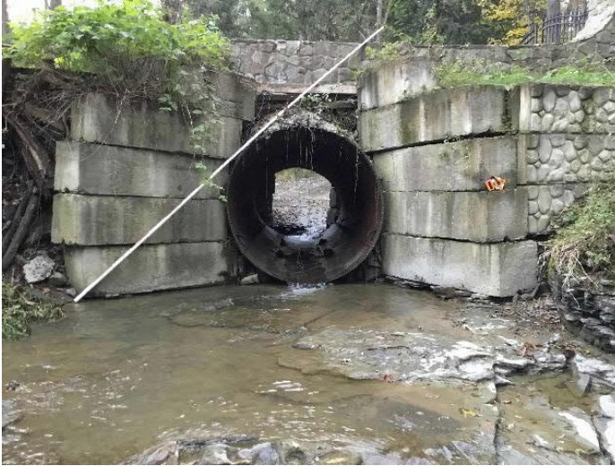
Private (Winery) Driveway off Allen Glen Road over Huntington Creek. Structure outlet. Note debris and plywood in place of headwall and severely misaligned wingwalls.
