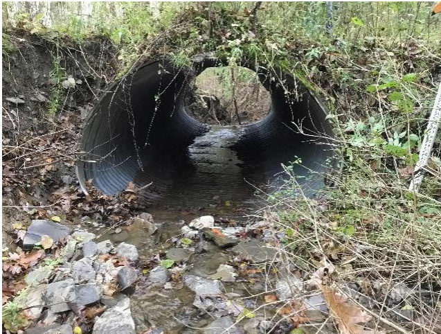
Private Driveway/Access Road off Carmichael Road over Tributary to Huntington Creek. Structure inlet. Note erosion on left side of structure.
