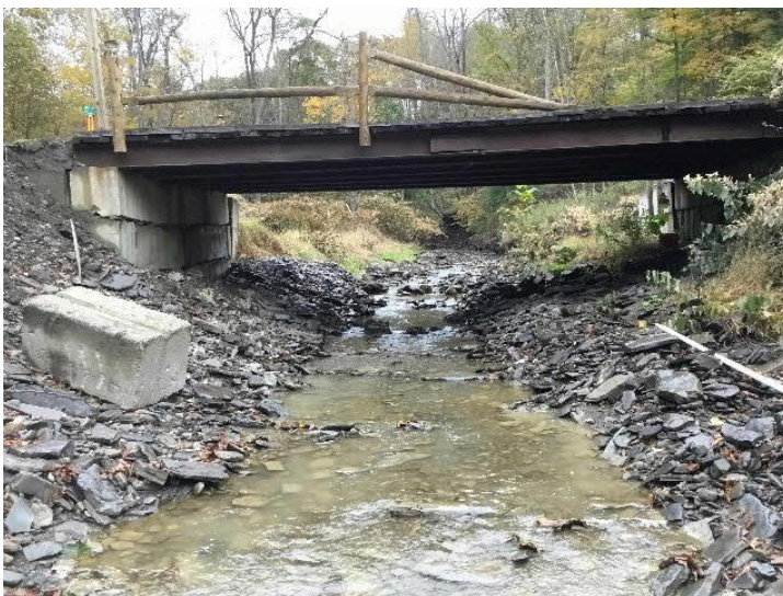
Private Driveway off Dean Street over Huntington Creek (downstream). Structure inlet. Note sagging abutment and displaced concrete waste block on left bank.
