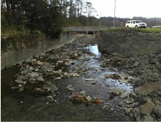
Huntington Creek channel downstream of Owego & Hartford Railroad bridge, looking toward Sheldon Guile Boulevard bridge. Note the concrete retaining walls lining the channelized stream.
