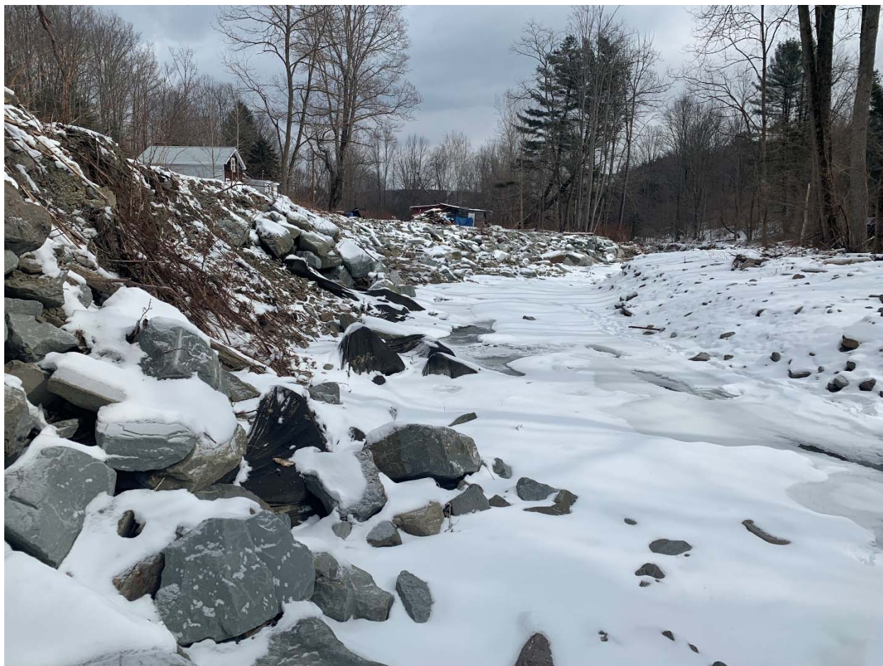
Figure 68. Failing rock bank protection at ApLo-3800. Photo taken March 7, 2019.
