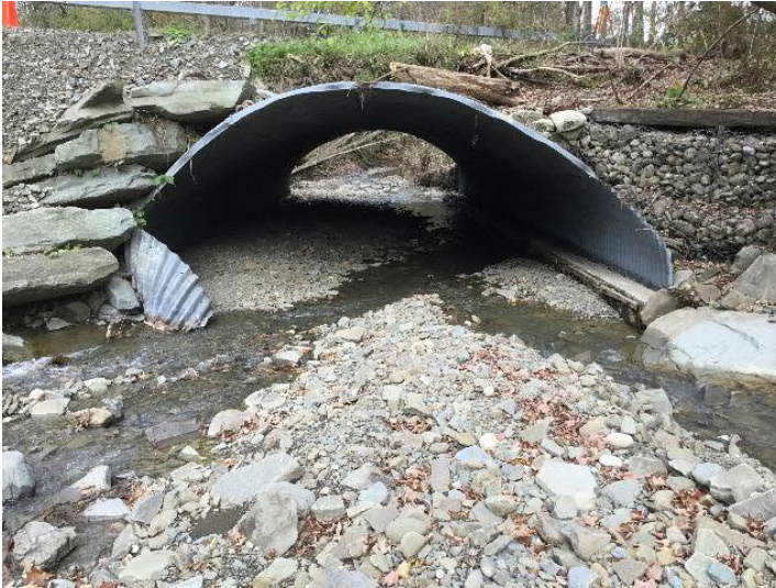
Long Creek Road over Long Creek (downstream of Section 4.4 crossing) - structure inlet. Note different wingwall materials on either side of outlet; exposed footings; and deformation of structure.
