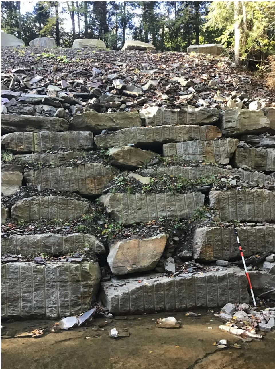
Figure 16. Stacked stone revetment used to protect Gaylord Road from being eroded by the creek. Photo taken October 19, 2018.
