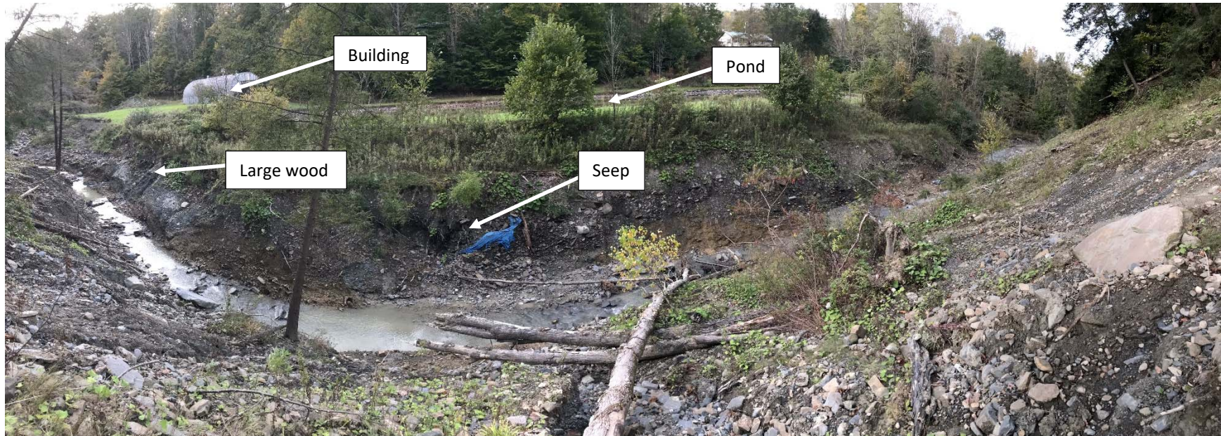
Figure 19. Panoramic view of incised channel and left bank with pond. Location of seep is noted. Blue article in photograph is a geotextile trapped within slumped bank material below the seep. Photo taken October 19, 2018.
