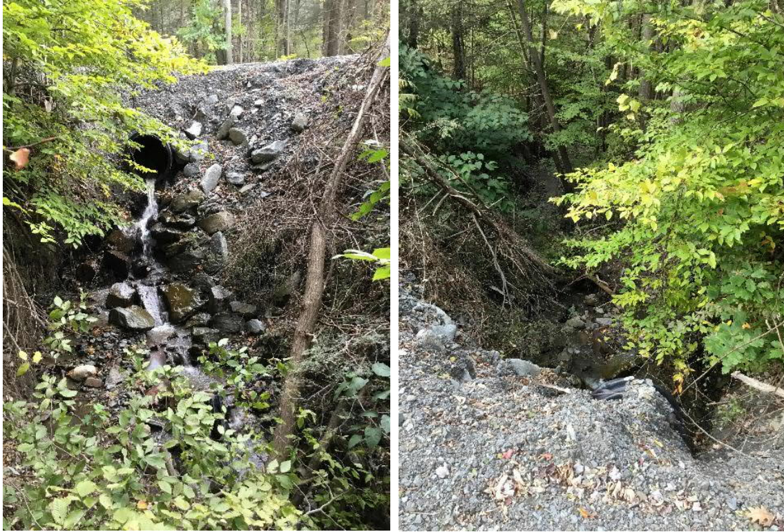
Chestnut Ridge Road over Deerlick Creek. Photograph of crossing outlet (left) and looking down at outlet from above (right). Note the large grade change, the perched outlet, and the erosion of the road evident in both photos.
