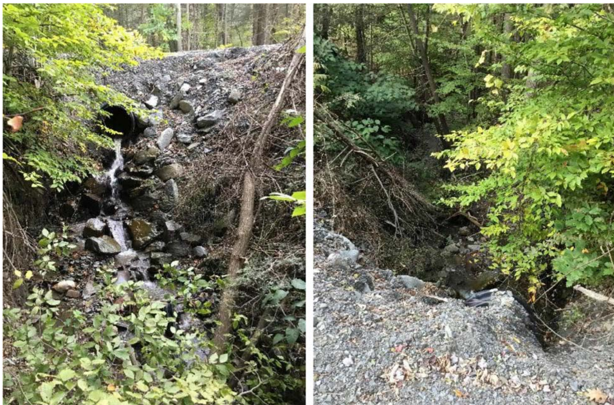
Figure 72. Chestnut Ridge Road crossing at ApDI-23700. Left image shows perched outlet. Right image is looking downstream along Deerlick Creek. Photo credit Fuss & O'Neill.
