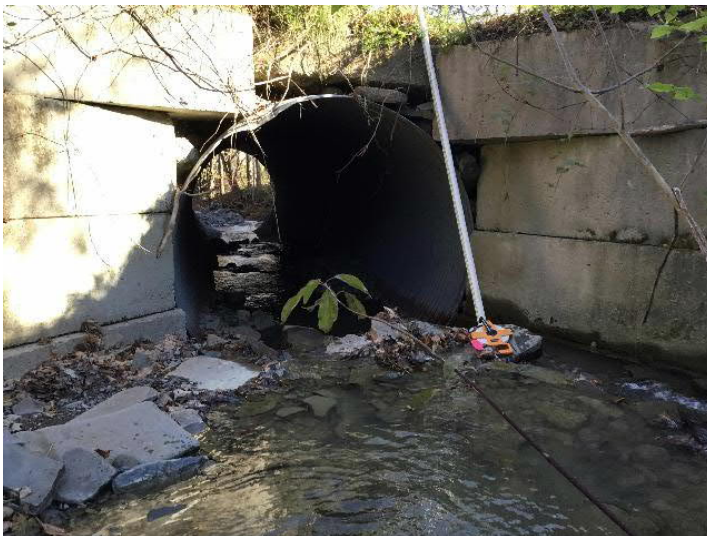
Card Road over Unnamed Tributary (Card Road Tributary) to Apalachin Creek - structure inlet. Note misaligned headwall, constriction in stream, and sharp bend in stream as it approaches the culvert.
