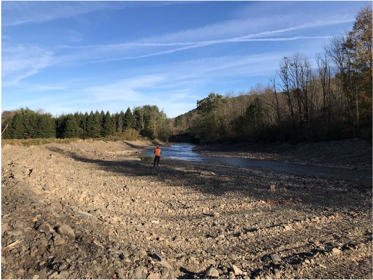
Figure 28. Looking downstream along Apalachin Creek near Ap-30000. Dredging and berming of the channel has resulted in an over-wide cross section, which reduces the channel's ability to transport sediment, resulting in deposition and more dredging. Furthermore, dredging is an activity that can have detrimental effects on upstream bed levels (i.e., causing headcutting), downstream hydraulics and sediment transport, aquatic habitat, and riparian species and therefore requires a permit. Berming can reduce instances of overbank flow and floodplain storage, thereby increasing downstream flood peaks. Photo taken October 19, 2019.
