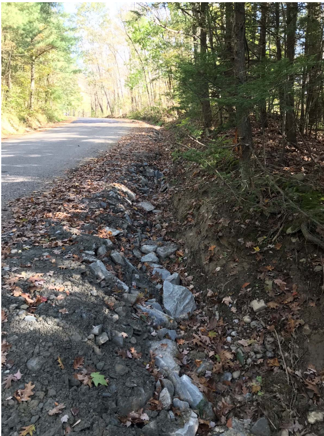
Figure 42. Eroding road ditch along Harnick Road delivering sediment to the Harnick Road tributary (project ApHa-2600). Photo taken October 19, 2018.
