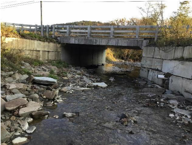
Pennsylvania Avenue over Unnamed Tributary to Apalachin creek – structure inlet. Note the relatively poor condition of the wingwalls and armoring.
