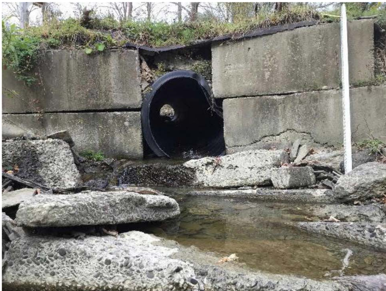
Figure 61. Outlet of perched and undersized Long Creek Road culvert carrying tributary to Long Creek at ApLo-12000. Photo credit Fuss & O'Neill.
