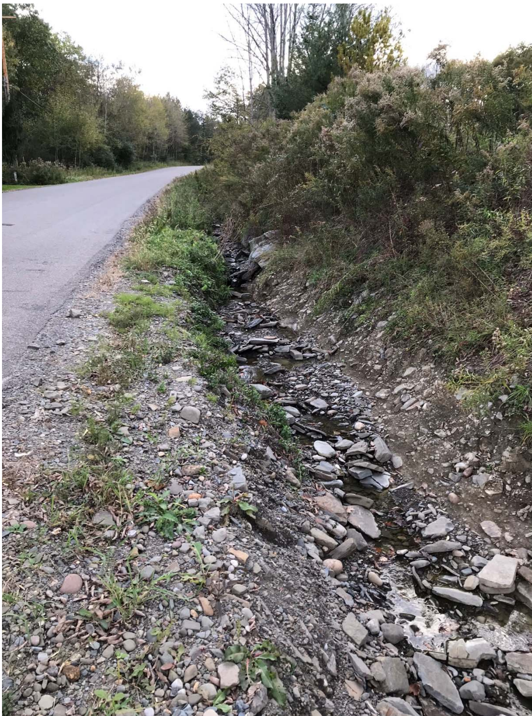
Figure 62. Incised road drainage ditch along Long Creek Road (ApLo-10800). Photo taken October 19, 2018.
