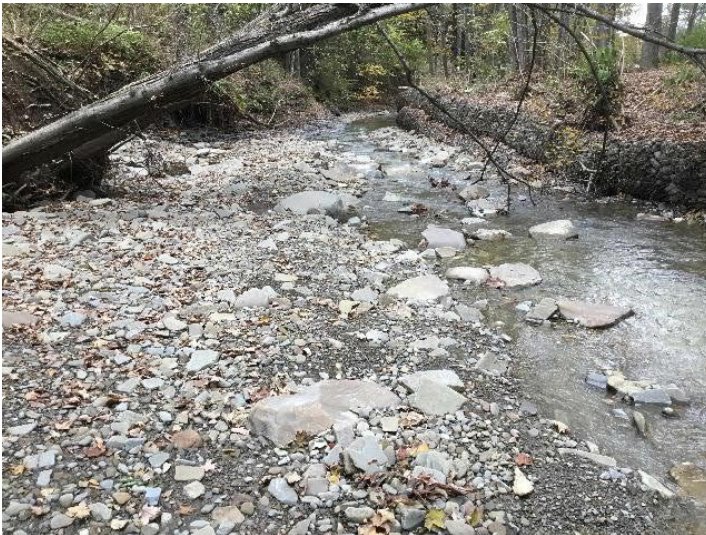
Long Creek Road over Long Creek (downstream of Section 4.4 crossing). Photograph of downstream channel. Note gabions retaining bank on right, eroded bank on left, and sediment deposition on left side of channel. Gabions farther downstream are undermined and leaning into stream.
