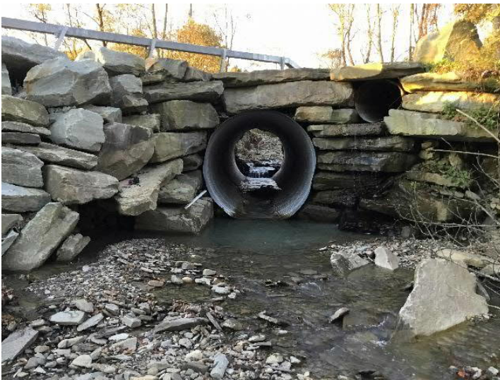
Fox Road over Unnamed Tributary to Apalachin Creek - structure outlet. Note unstable wingwall with large void at base, at left side of photo.
