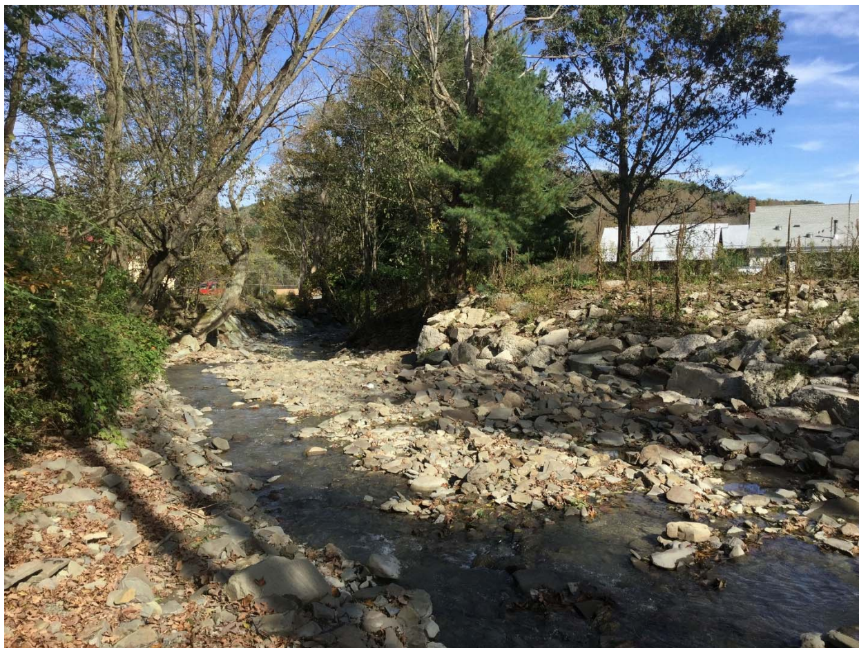
Figure 9. Lower reach of the unnamed tributary along Fox Road showing rip rap placed on the channel banks to protect infrastructure and private property. Photo taken October 19, 2018.
