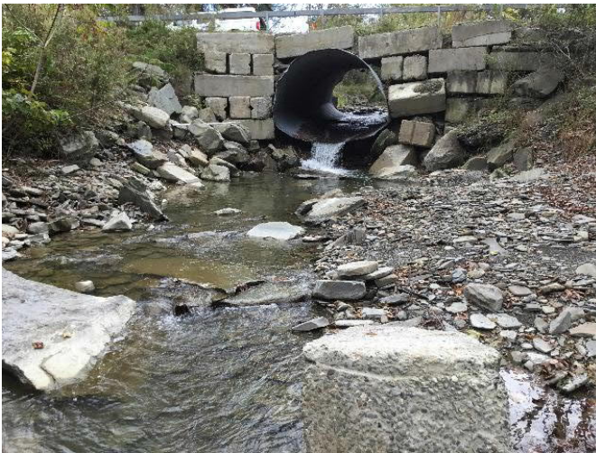
Gaylord Road over Unnamed Tributary to Apalachin Creek (at Little Hill Road) - crossing outlet. Note unstable headwalls and perched, undermined outlet of culvert.
