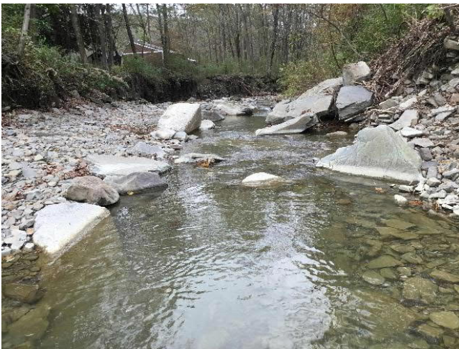
Gaylord Road over Unnamed Tributary to Apalachin Creek (at Little Hill Road). Eroded channel banks downstream of structure threaten residential property on river left.
