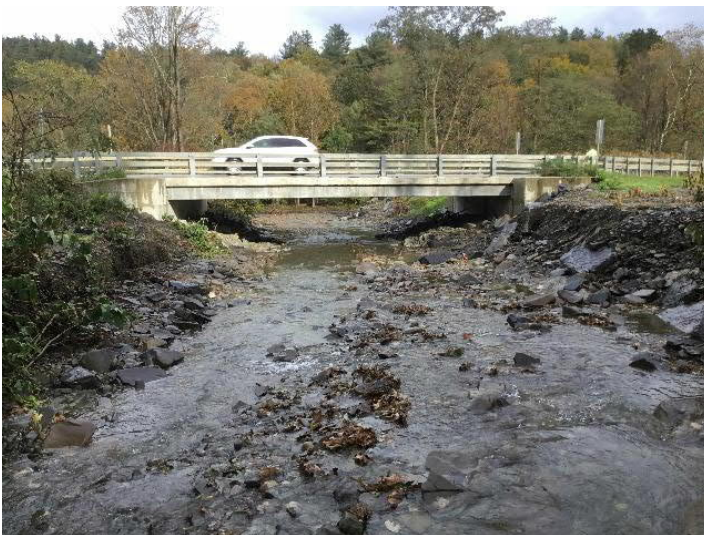
Pennsylvania Avenue over Long Creek - structure inlet. Note the bank erosion on the upstream side of the crossing and scour of the embankment at the crossing structure.
