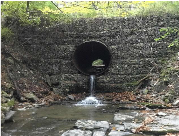
Beach Road over Unnamed Tributary to Deerlick Creek - structure outlet. Note that culvert is perched 4.6 feet above streambed. Downstream channel has been scoured to bedrock due to high-velocity flows exiting culvert and limited sediment supply (likely due to constriction).
