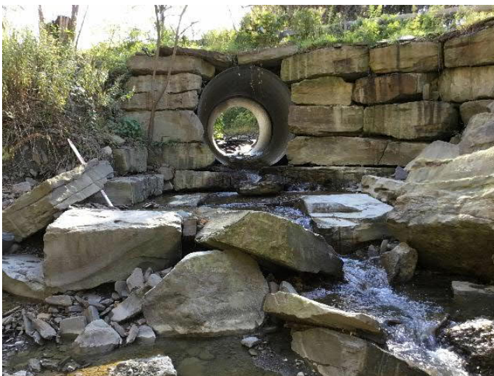
Gaylord Road over Unnamed Tributary to Apalachin Creek (upstream of Section 4.6 crossing) - structure outlet. Note that outlet is perched. Also note headwall in poor condition and displacement of joint inside of culvert pipe.
