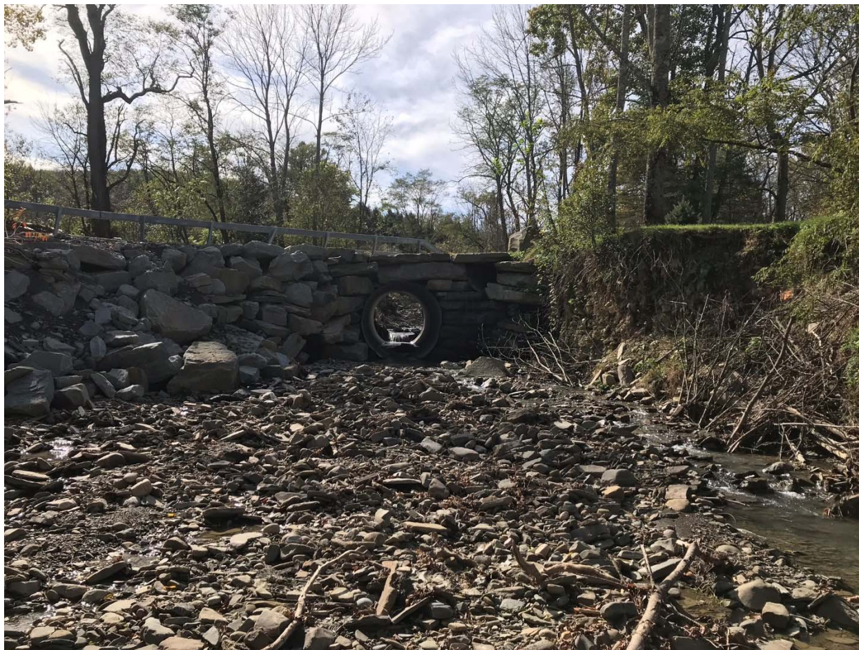
Figure 36. Downstream headwall at ApFo-1300. Photo taken October 19, 2018.
