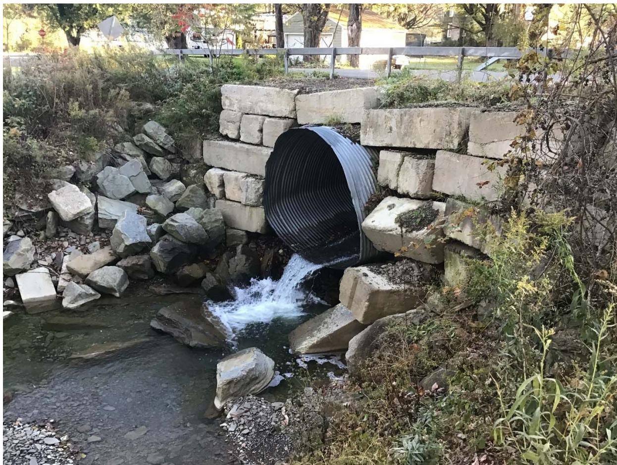
Figure 60. Outlet of perched and undersized culvert at ApGa-600. Photo taken October 19, 2018.
