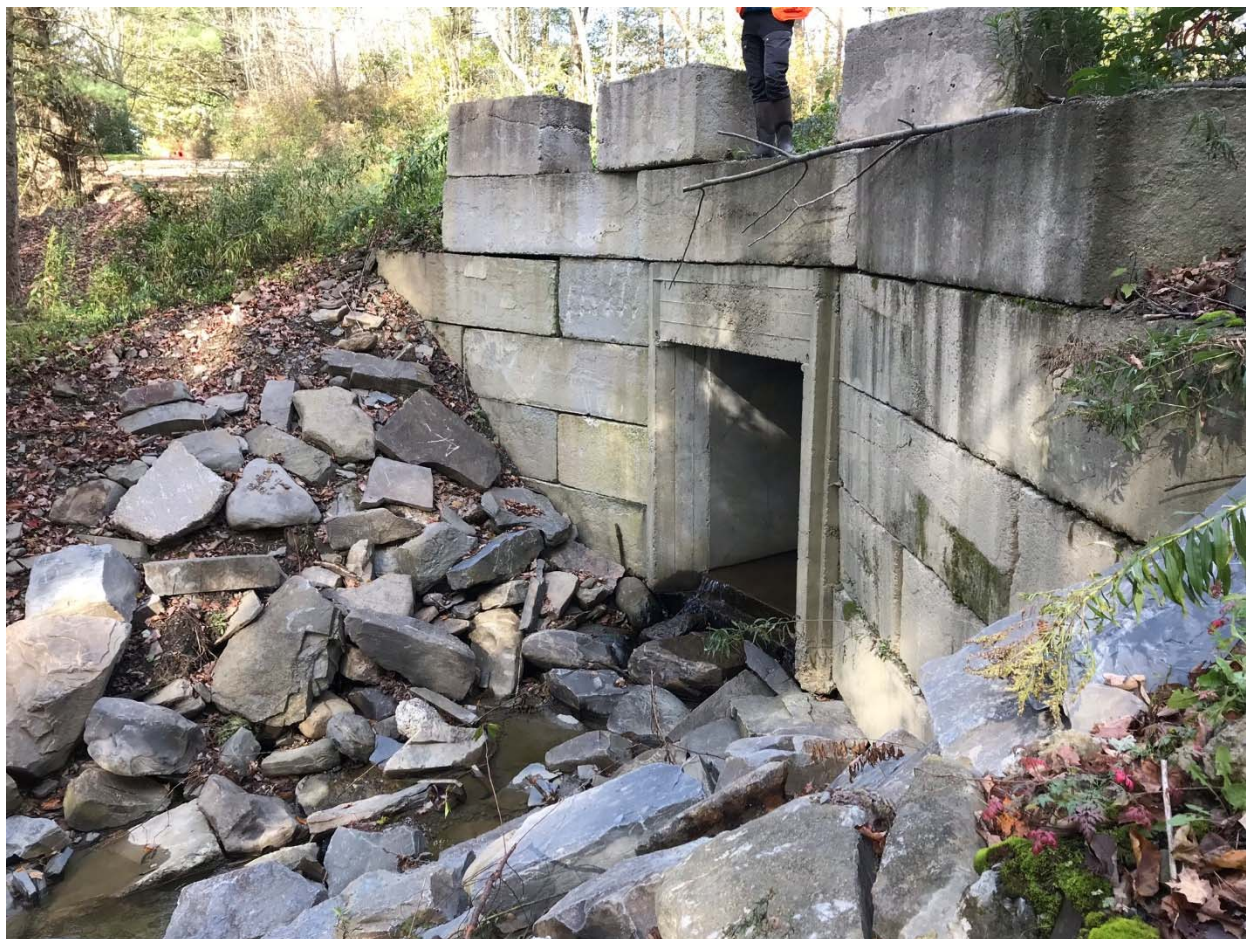
Figure 40. Undersized box culvert at Apha-5800. Photo taken October 19, 2018.
