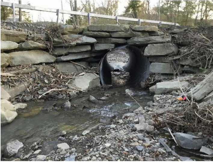
Fox Road over Unnamed Tributary to Apalachin Creek - structure inlet. Note misaligned headwall, constriction in stream, and sharp bend in stream as it approaches the culvert.
