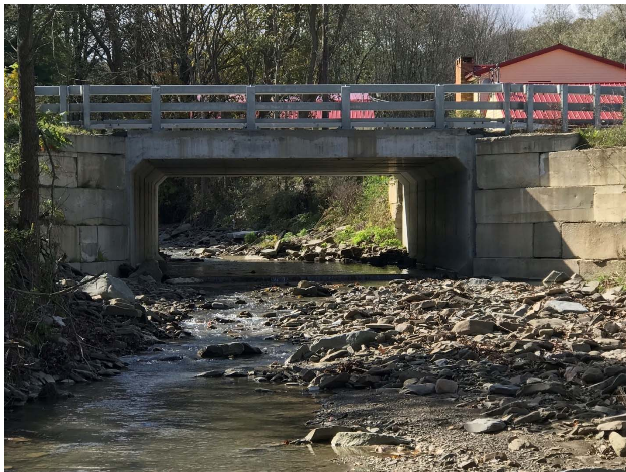
Figure 38. Looking upstream at Pennsylvania Avenue crossing ApFo-600. Concrete bed is slightly perched. Photo taken October 19, 2018.
