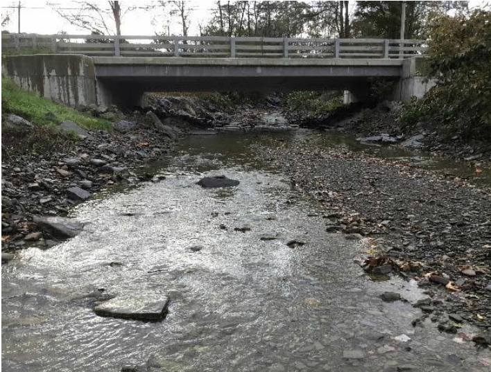
Pennsylvania Avenue over Long Creek - structure outlet. Note the erosion of the embankment and armoring below and immediately downstream of the crossing structure.
