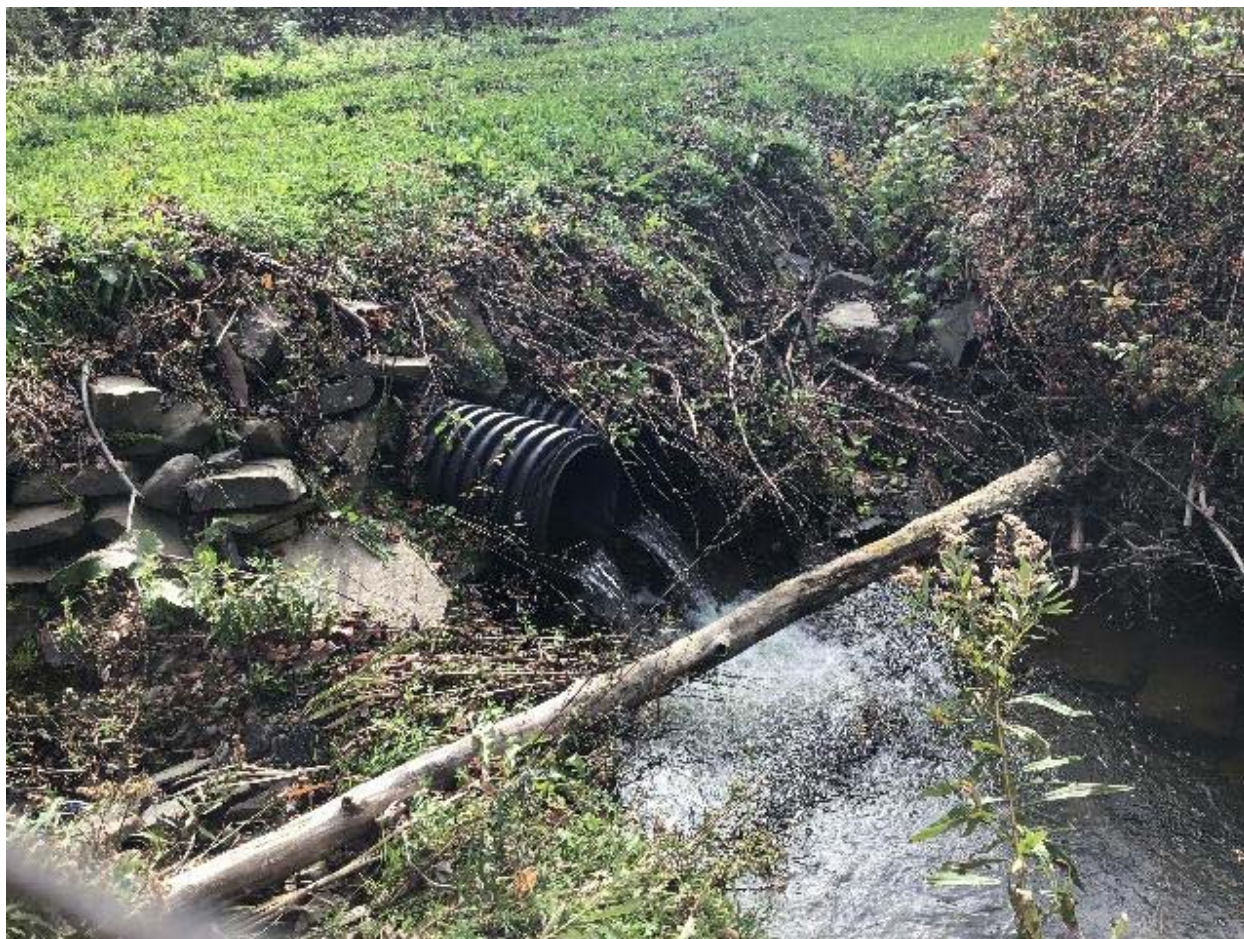
Figure 73. Twin undersized and perched culverts at ApDI-21100. Photo taken October 18, 2018.
