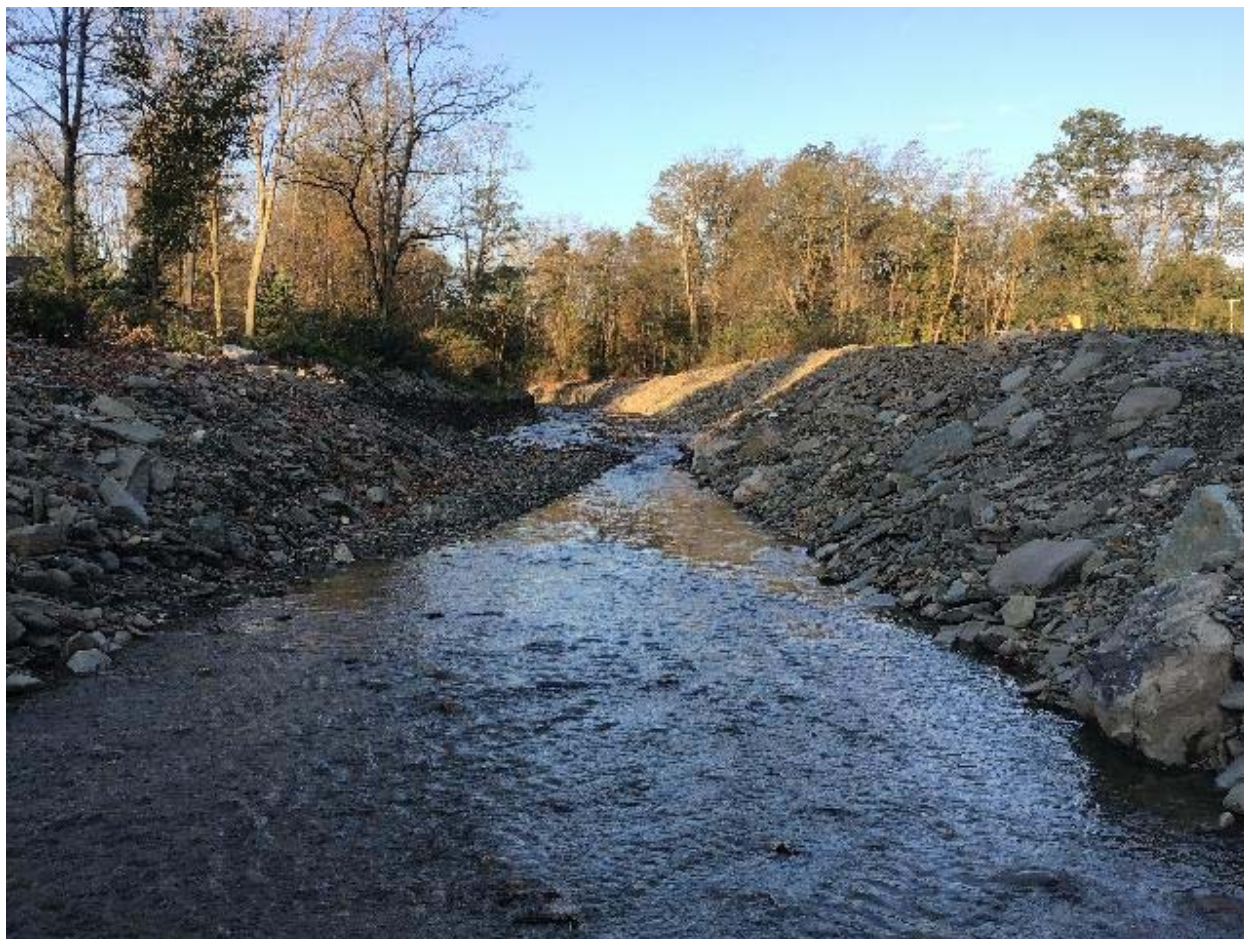
Figure 77. Deerlick Creek at ApDI-500. Channel has been straightened and dredged, minimizing potential access to former floodplain. Photo taken October 18, 2018.
