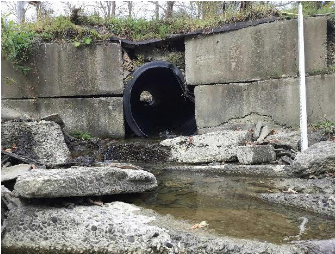
Long Creek Road over Unnamed Tributary to Long Creek - structure outlet. Note deformed outlet of pipe; misaligned wingwalls; vertical hydraulic drop downstream of outlet, and eroding soil and exposed geotechnical fabric supporting the road above the culvert.
