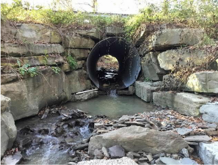
Card Road over Unnamed Tributary (Card Road Tributary) to Apalachin Creek - structure outlet. Note that outlet is perched.
