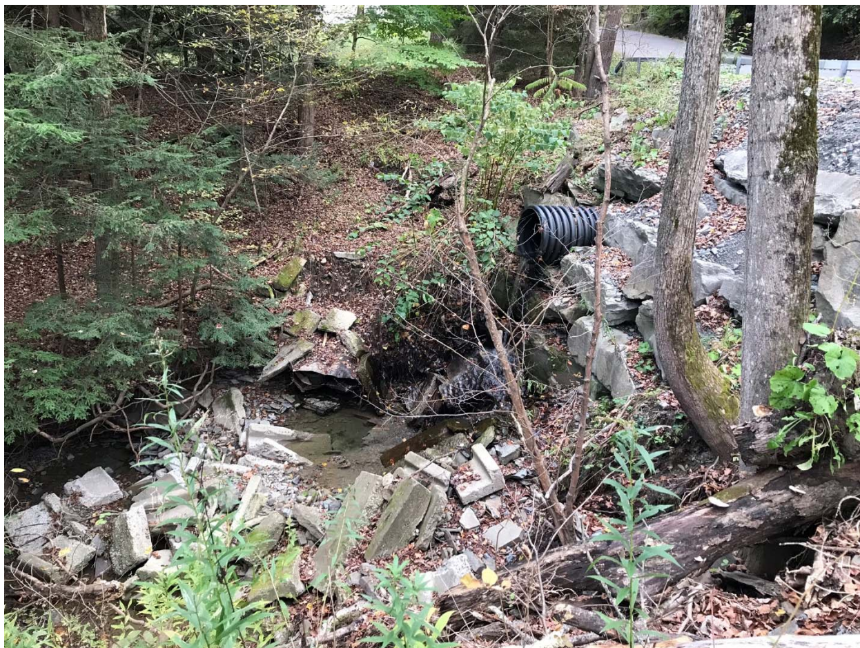
Figure 66. Perched culvert outfall at ApLo-9200. Photo taken October 19, 2018.
