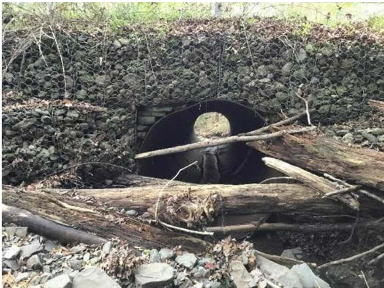
Figure 75. Undersized and blocked Beach Road tributary culvert inlet at ApDI-8900. Photo taken October 18, 2018.
