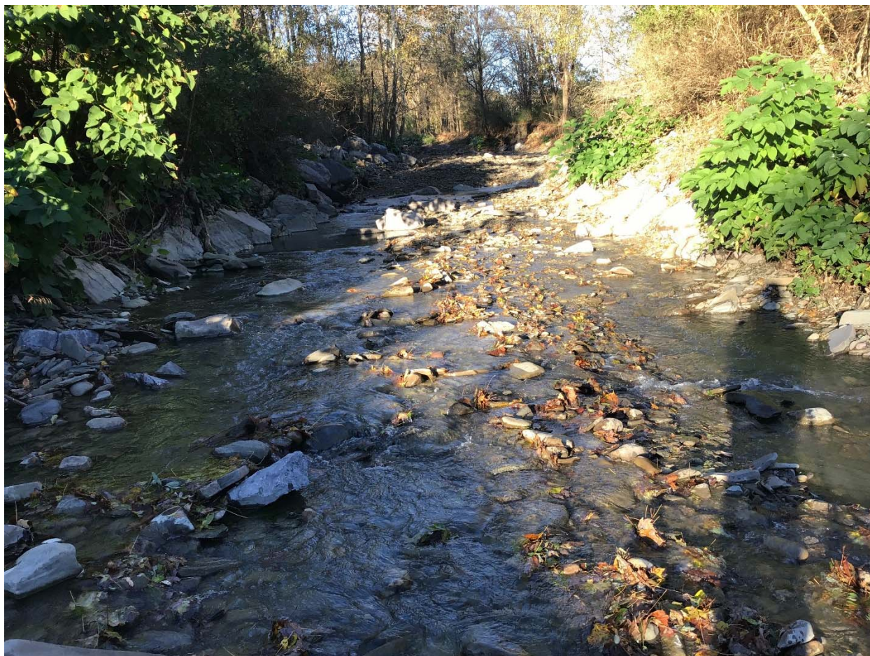
Figure 71. Long Creek channel at ApLo-400. Channel has been straightened and dredged, minimizing potential access to former floodplain. Note rock bank protection and the presence of the invasive Japanese knotweed on the banks. Photo taken October 18, 2018.
