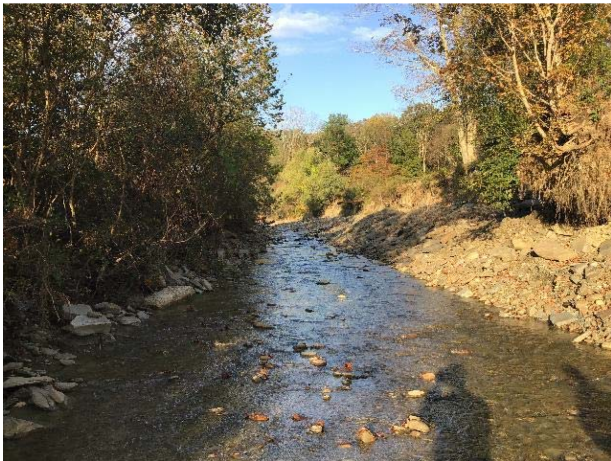
Figure 76. Deerlick Creek at ApDI-1500. Channel has been straightened and dredged, minimizing potential access to former floodplain. Photo taken October 18, 2018.
