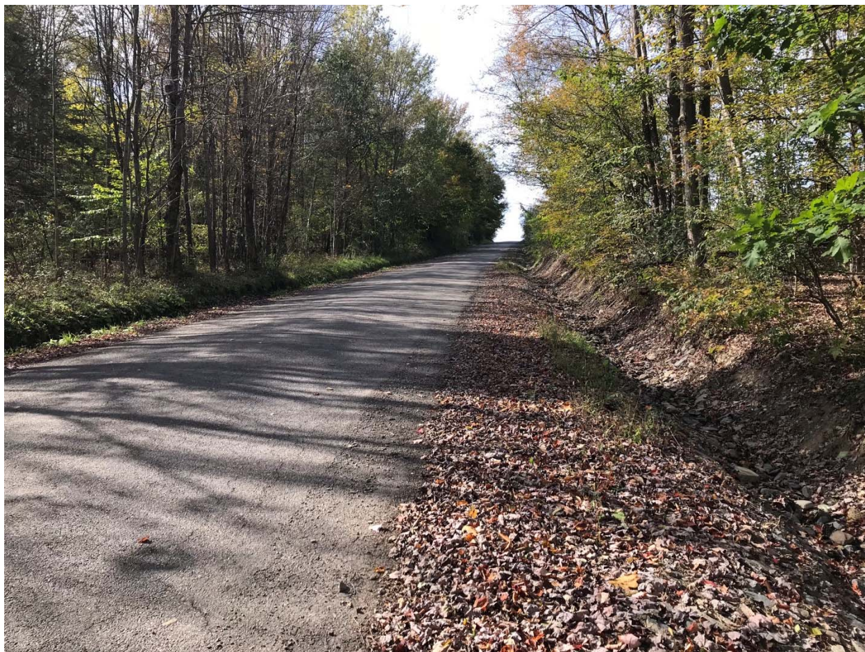
Figure 35. Incised road ditch along Fox Road (ApFo-4000). Photo taken October 19, 2018.
