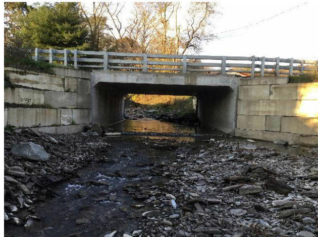
Pennsylvania Avenue over Unnamed Tributary to Apalachin creek – structure outlet. Note the slightly perched invert at the structure outlet.
