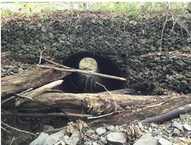
Beach Road over Unnamed Tributary to Deerlick Creek - structure inlet. Note debris blocking inlet. Gabions behind debris near culvert base are partially or fully collapsed.
