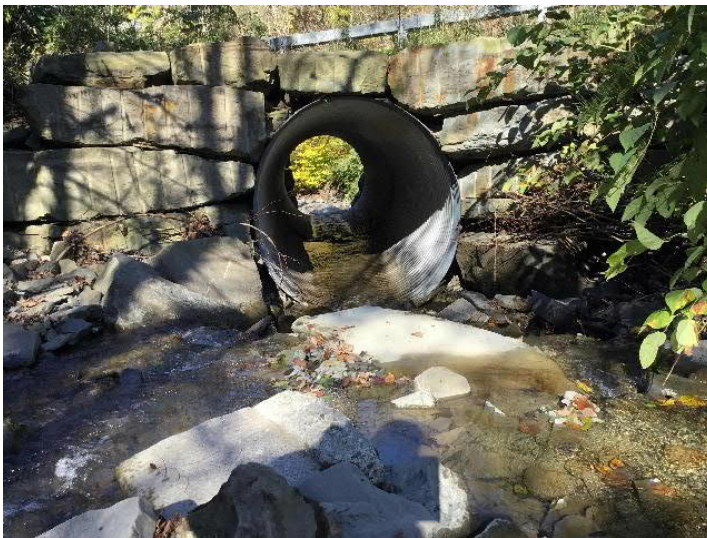
Gaylord Road over Unnamed Tributary to Apalachin Creek (upstream of Section 4.6 crossing) - structure inlet. Note misaligned headwall and constriction of stream.
