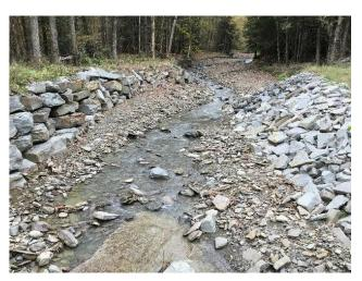
State Line Road over Unnamed Tributary at Briggs Hollow – upstream of crossing. Right stream bank is eroding at upstream end of stone revetment.
