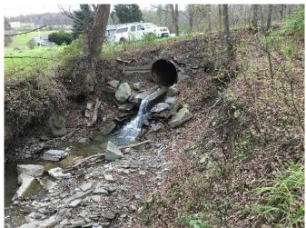
Briggs Hollow Road over Unnamed Tributary at Briggs Hollow - crossing outlet. Note steep drop from culvert, eroded channel downstream, and sloughing of soil from road embankment.
