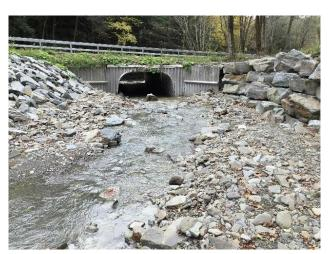
State Line Road over Unnamed Tributary at Briggs Hollow - crossing inlet. Note stone revetment placed upstream of the inlet when the crossing structure was replaced following washout in 2011.
