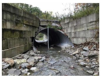
Lower Briggs Hollow Road over Unnamed Tributary at Briggs Hollow - crossing inlet. Note gaps between wingwalls/headwall and pipe that may allow seepage, and misaligned wingwall blocks.
