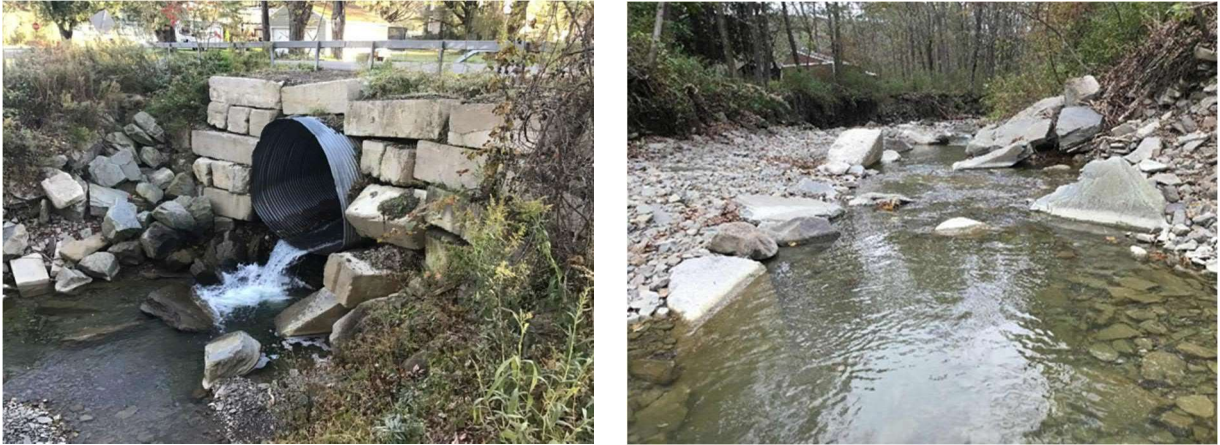
Figure 1. Downstream side of the existing Gaylord Road culvert showing the perched outlet and poor condition of the concrete block headwall (left) and severe bank erosion on the left bank downstream of the culvert that is threatening residential structures (right).
