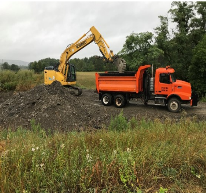
Above: Removal of sediment in the upper SVE high school sediment basin
